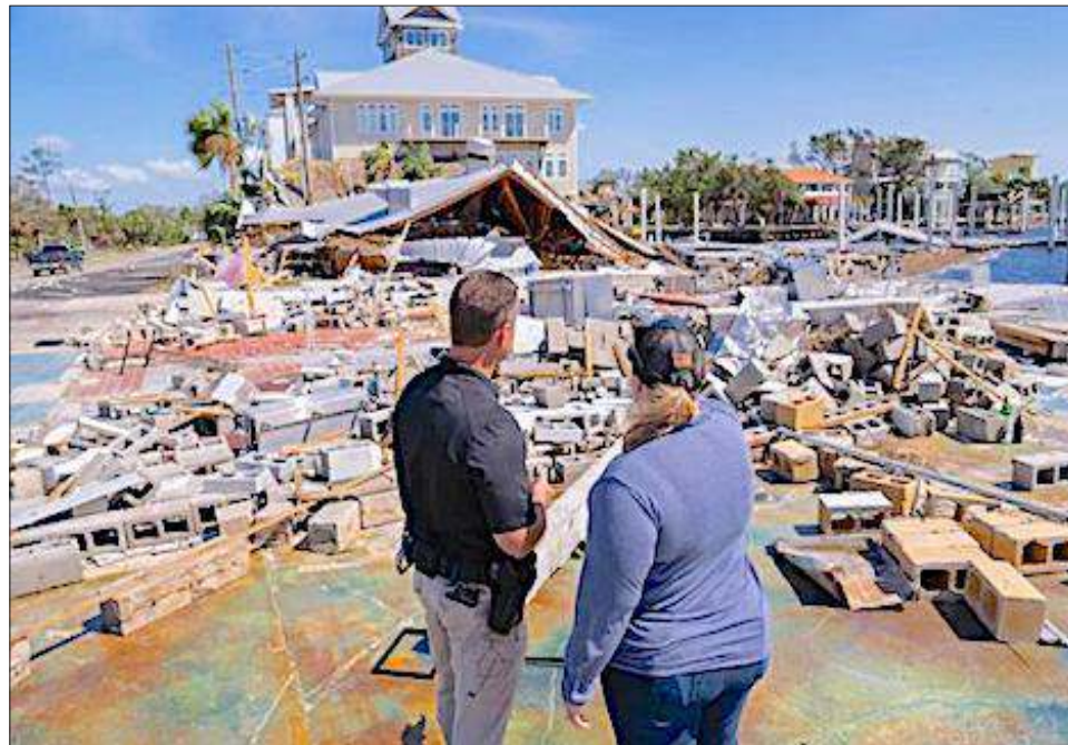
Rep. Cammack tours damage in Florida's Third Congressional District the day after Hurricane Helene made landfall.
